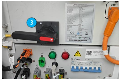
Figure 5-10: Disconnect the PCS circuit breaker
