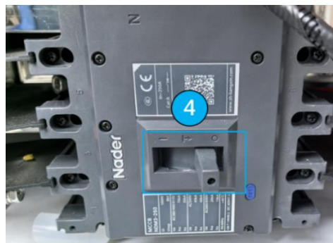
Figure 5-11: Disconnect MCCB QF0 switch
