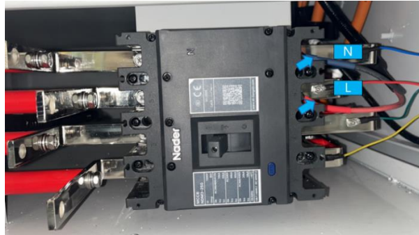
Figure 4-38: Auxiliary power cable position (EU&AU version)
