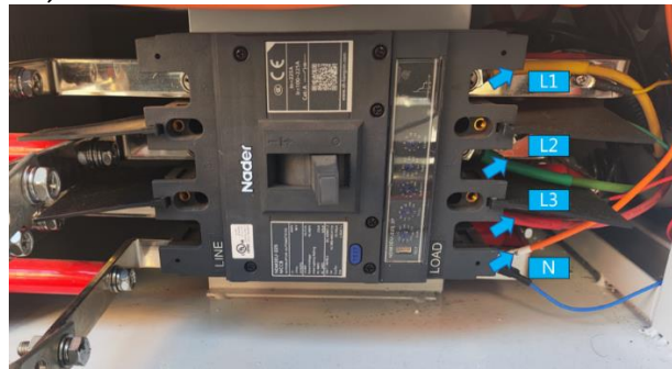
Figure 4-39: Auxiliary power cable position (NA Version)
