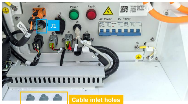
Figure 4-55: auxiliary power connection position in control box
