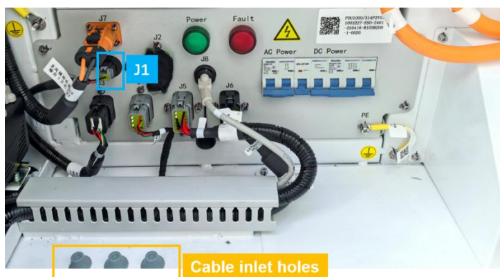
Figure 4-41: Control box J1 interface position
