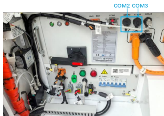
Figure 4-47: Diagram of PCS parallel communication interface
