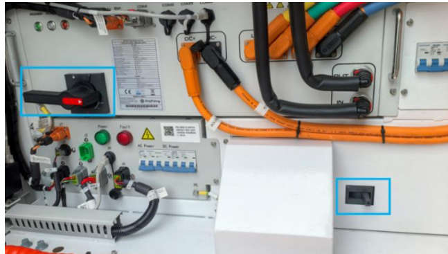
Figure 5-1: MCCB and PCS handle position
