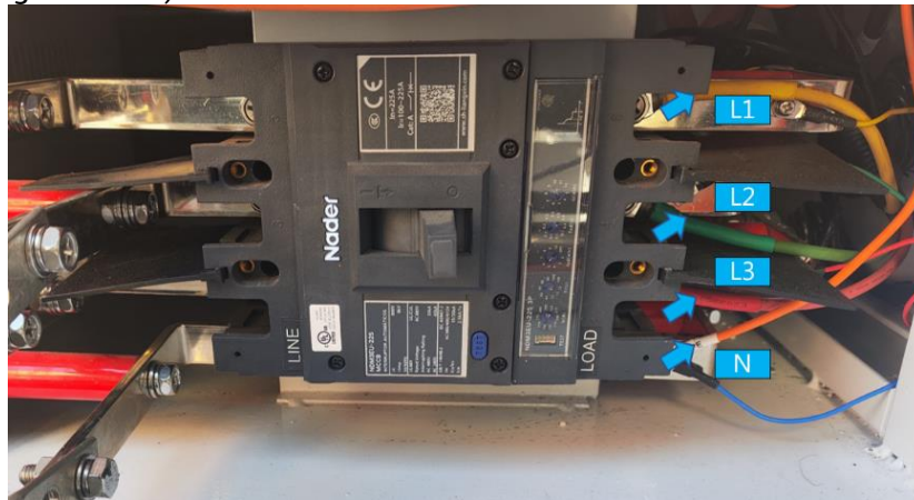
Figure 4-52: Auxiliary power cable position (NA Version)
