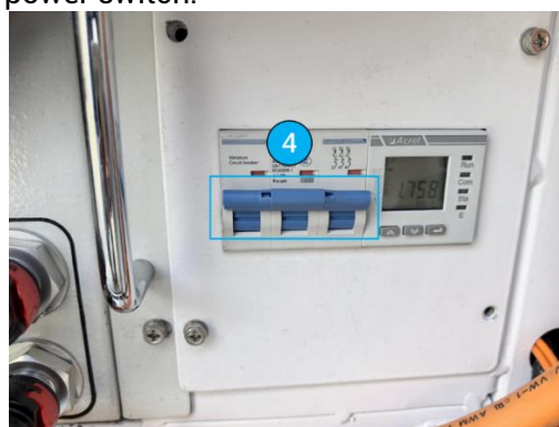
Figure 5-5: Turn on liquid cooling power switch
